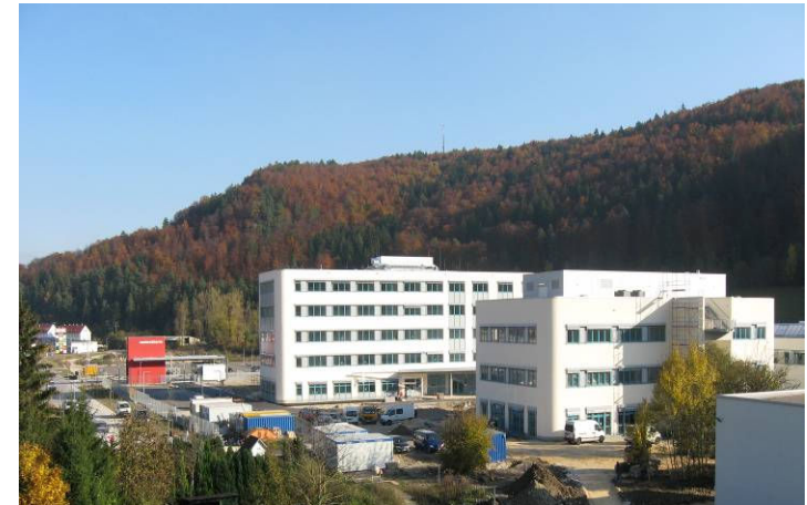
New offices in Blaubeuren are near completion
