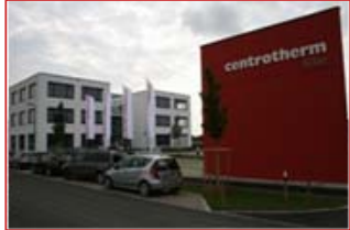
CT Sitec, Burghausen
